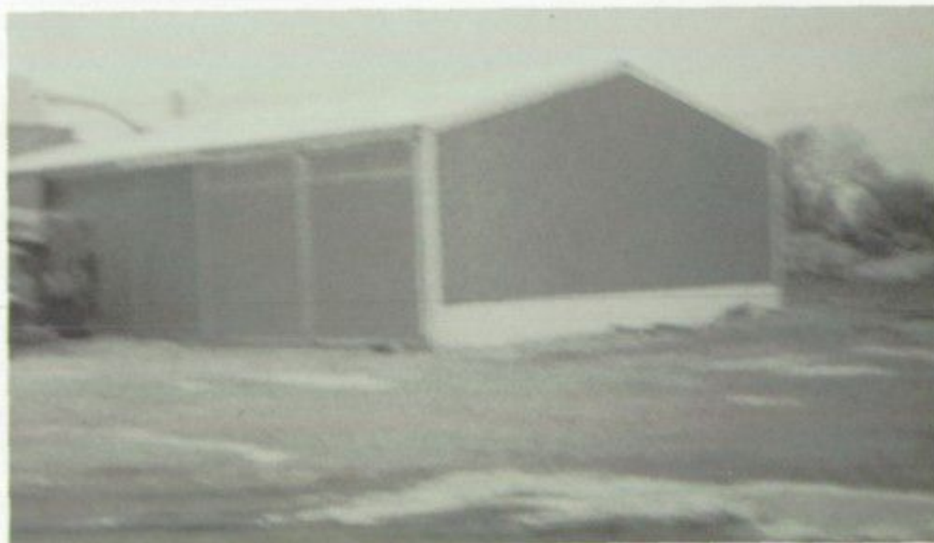
New Addition to Kaple Lumber Company
