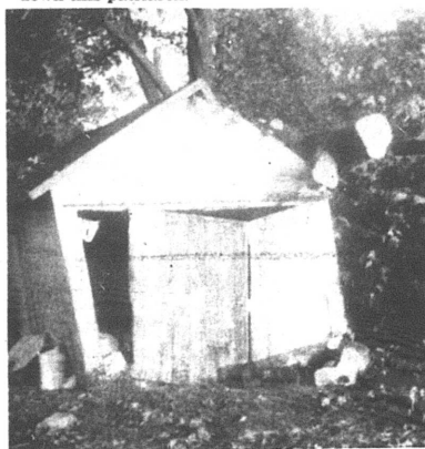
After upper limbs were sawed off, passersby could see what storm did to garage of Richard Roll, 79 Plymouth street.
