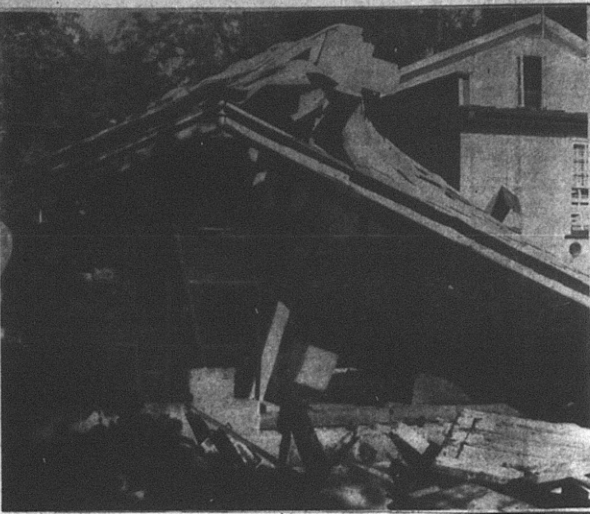
ALL THAT WAS LEFT of frame building at 39 Bell street after Monday's explosion. Roof was raised 30 feet, eyewitnesses said, by force of blast. Roy Carter's residence, windows broken, is visible at the right.
