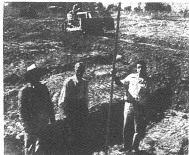
Bulldozers in tandem tackled the excavating work. Here, left to right, George Mittenbuhler, Ernest Davis and Leo Barnes stand in the core trench of the dam.
