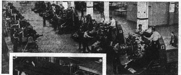
A Part of a nationwide synchronization of America's industrial forces to produce this great plane is the world's largest factory, Dodge Chicago Plant, Division of Chrysler Corporation, exclusively devoted to mass production (above) of 2200 h.p. Wright Cyclone engines to power the Superfortress.
