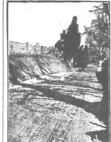
Good Road in Southwest.
