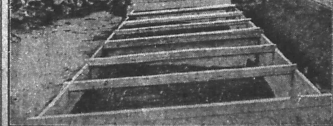
In a Dry Spot in the Garden Excavate for a Depth of Two Feet or More for Your Cold Pit.
