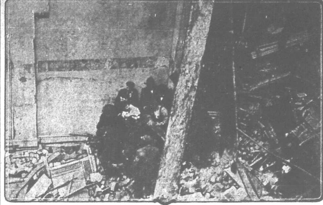
The building of the St. Louis Feed company of St. Louis was demolished when a portion of a seven-story wall of the burned Missouri Athletic club toppled over on it.
